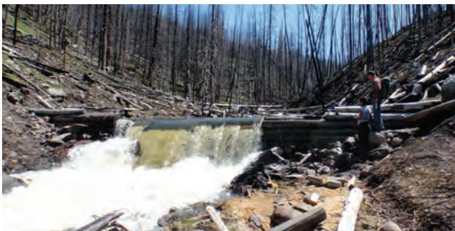
This barrier on East Fork Specimen Creek prevents nonnative fish from invading the restoration area.
