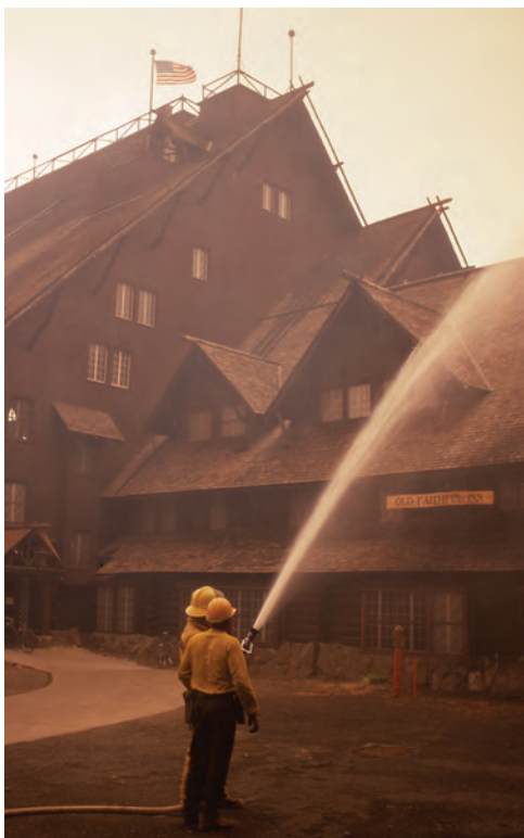
Firefighters worked to prevent historic structures like the Old Faithful Inn from burning.
