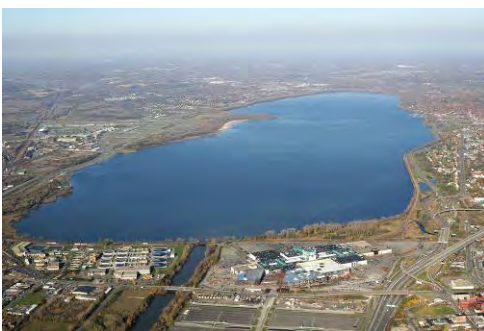
SMU 8 is located in the center of the lake in greater than 30 feet of water.
