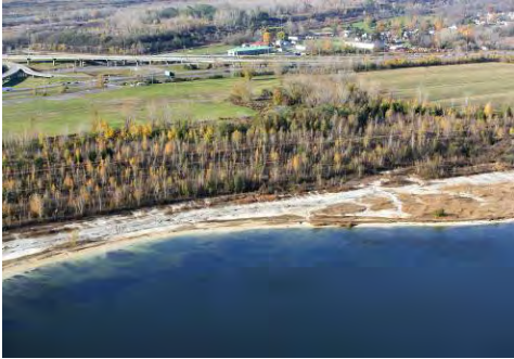
This exposed Solvay Waste along the shoreline of Wastebeds 1-8 will be addressed as part of the habitat enhancement activities discussed in this section.
