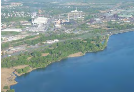
The Wastebed B/Harbor Brook IRM barrier wall will be installed near the shoreline in this area.
