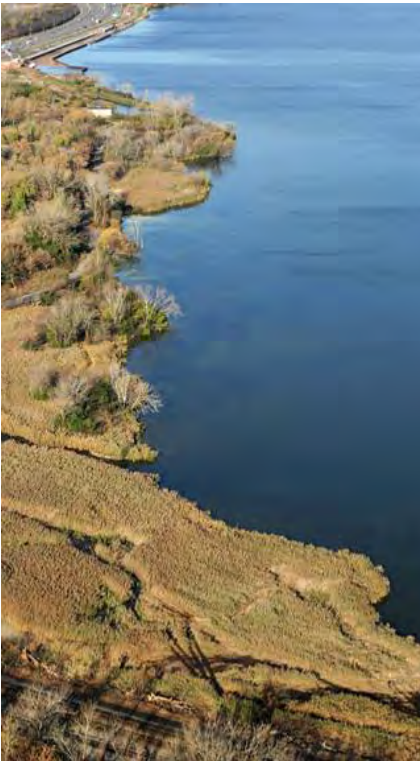
Remediation Area D is located adjacent to the Wastedbed B/Harbor Brook site.
