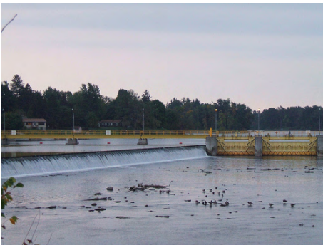
The Phoenix Dam, located in Phoenix, New York, controls the level of Onondaga Lake.
