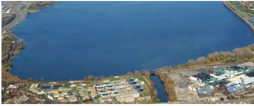
Remediation Area E (SMU 6 and 7) is located between Harbor Brook and Ley Creek on the eastern shoreline of the lake.
