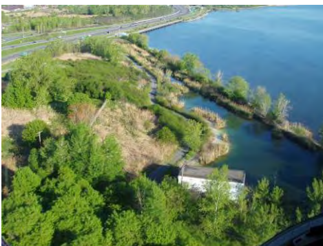
The East Flume is a water conveyance system located along the southern shoreline of Onondaga Lake.
