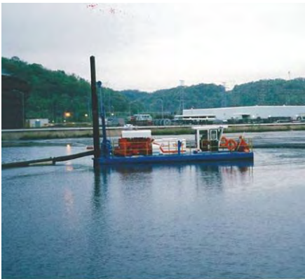
Hydraulic dredging operation
