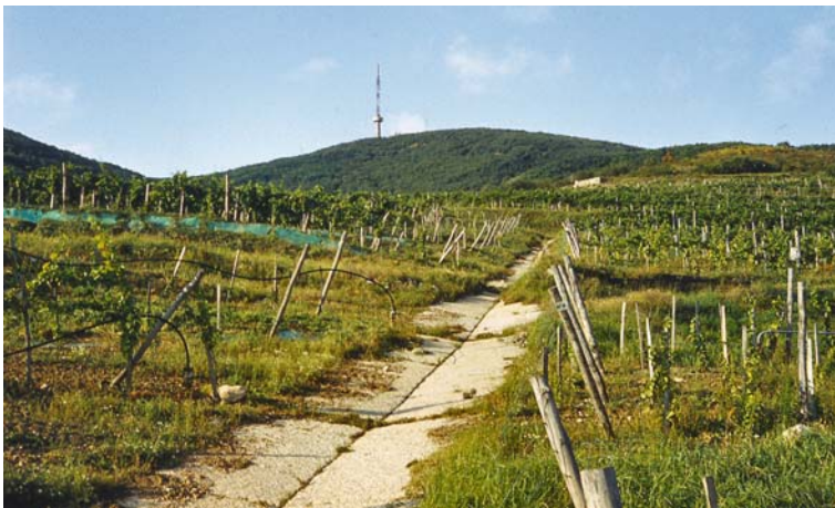
Plate 7.6 A concrete road also functioning as a drainage ditch between terraced irrigated vineyard plots, in the vicinity of Tarcál (Tokaj-Hegyalja Region) (Csorba 1985)
