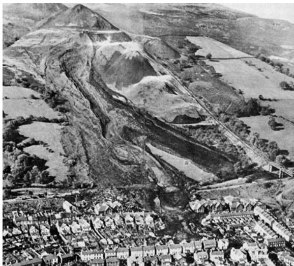
Plate 10.3 The waste tip at Aberfan slumped on 21 October 1966 (Bolt et al. 1975)
