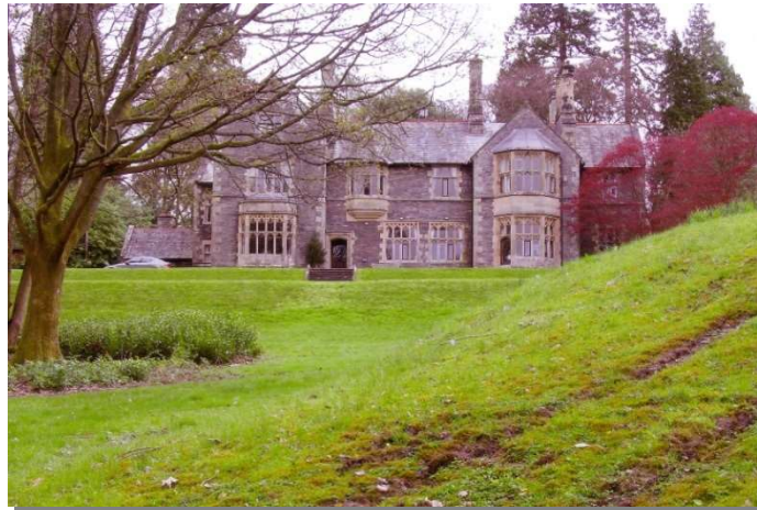
Figure 11.II.12 The west-facing side of Fallbarrow Hall (spring 2018). The land on this side naturally slopes down to Lake Windermere, so two terraces were created to give level areas beside the hall. More recent landscaping (mound on the right) was undertaken to give privacy between the occupants of the log cabins and the tenants of the hall. The round bed indicated on the Ordnance Survey map 1897 is still present (on the left).
