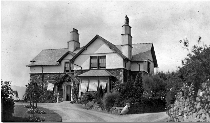
Figure 11.III.27 Lindeth Fell — photograph c. 1913. Houses built by the local builders, Pattinsons, were frequently of a similar style combining white roughcast, local stone, and Westmorland slate, together with numerous gables and round chimney stacks.
