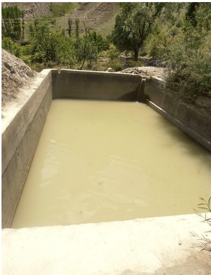
Exhibit 27: Water storage tank at village in Ghulmat valley
