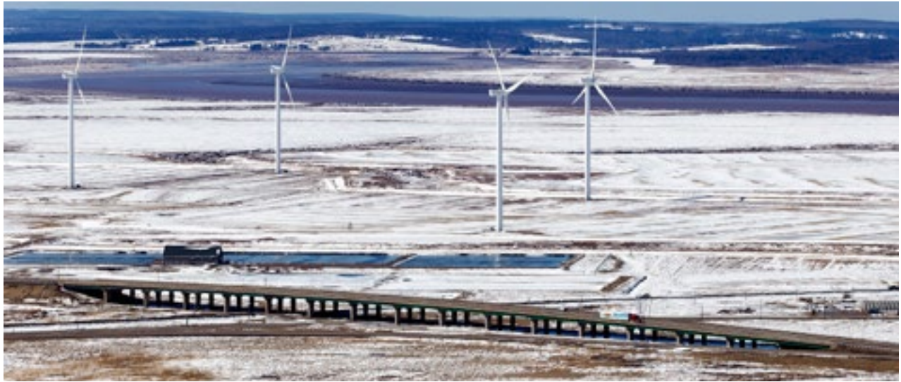
Wind turbines on the Cumberland Marshes along the Trans-Canada Highway north of Amherst, take advantage of the near constant winds that channel through this lowland area from the Cumberland Basin and Bay of Fundy. PHOTO: CNS (Len Wagg)
