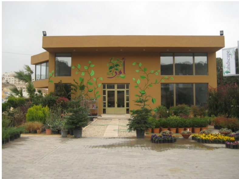
Figure 5: Area to be developed into a water-wise show area at Ur Garden
