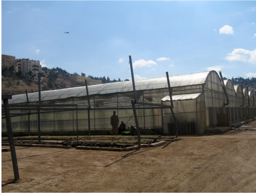
Figure 1: Multi-span greenhouse at al-Qadisiyya Nursery
