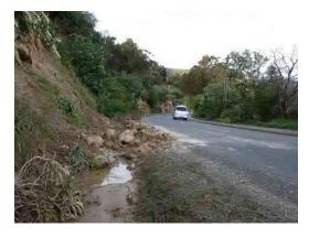
Discharges of storm water from roads is observed damaging banks on both sides of roads.
