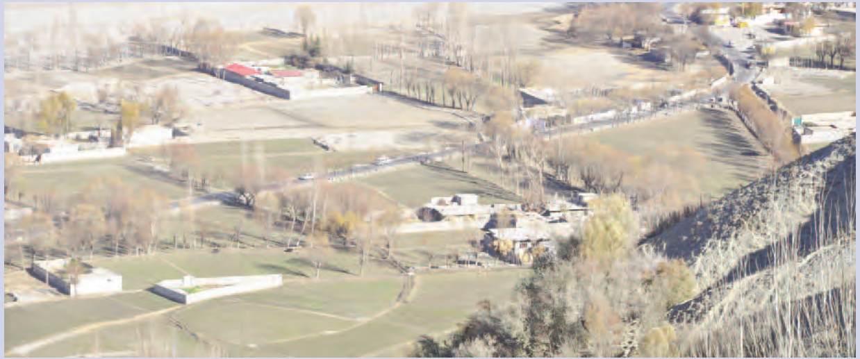
Exhibit 3.29: Construction on a Riverbank
