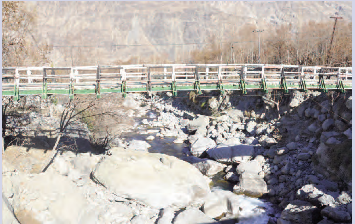
An old footbridge over the Kargah Nullah
