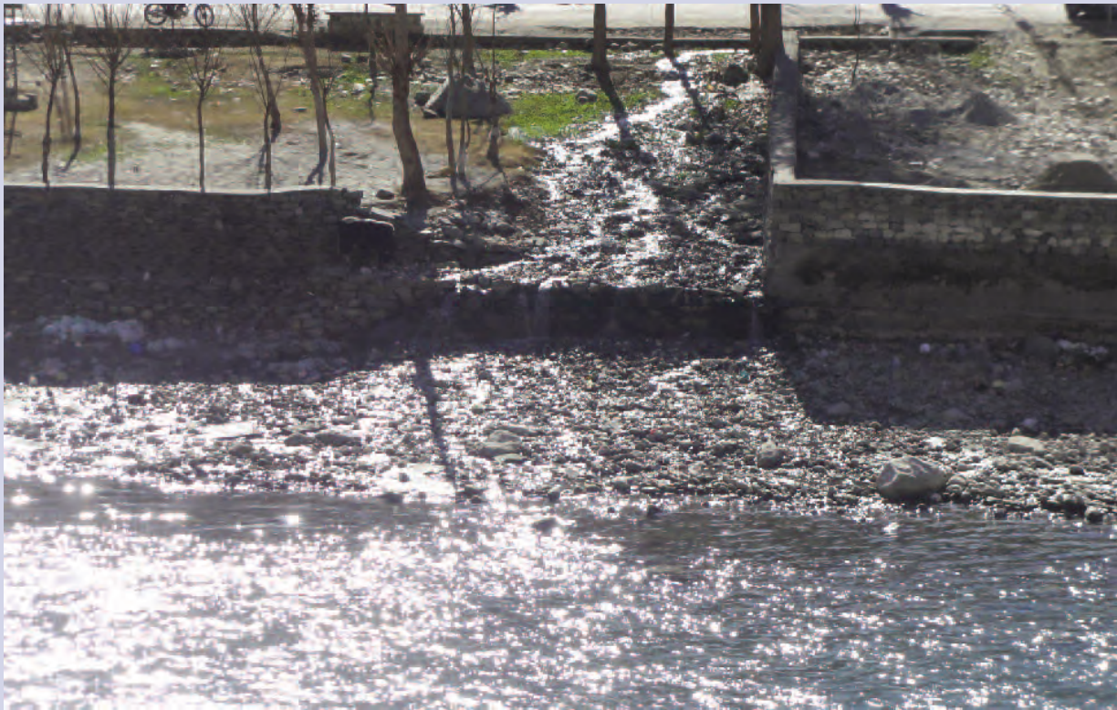
A stream of untreated effluent from a drain flowing into the Gilgit River.
