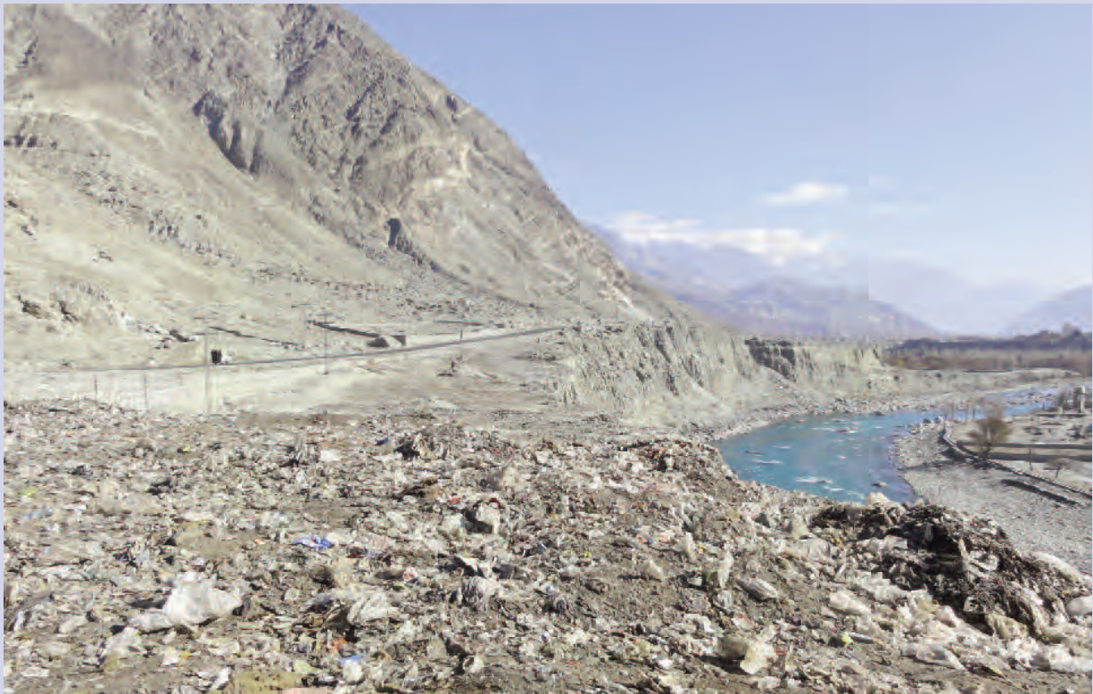
A large waste dump in Konudas which falls into the river
