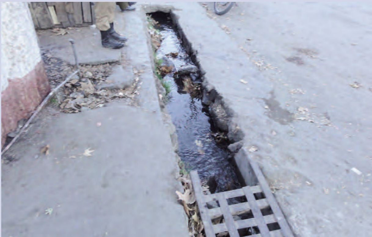
An open drain next to the footpath.
