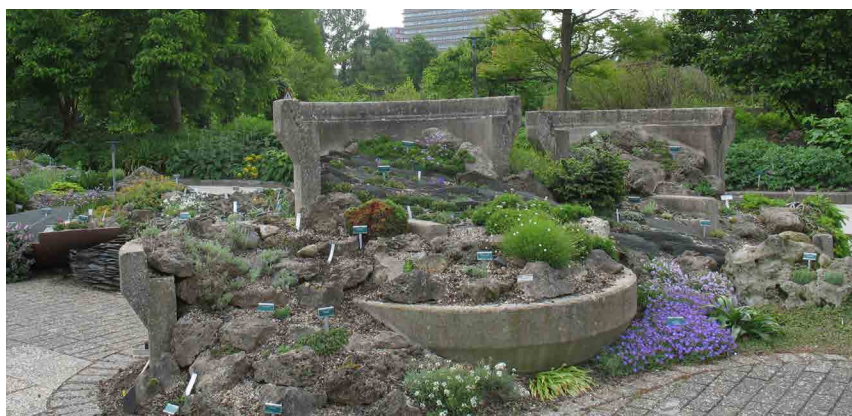
Concrete sewer pipes sawn in half form the main structure of a tufa bed.
