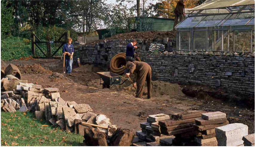
The first broken-concrete retaining wall in the garden being built in 1989.
