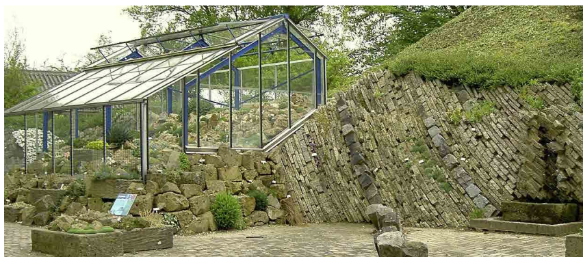
The tilted strata retaining wall and alpine house. Photo by Wiert Nieuman
