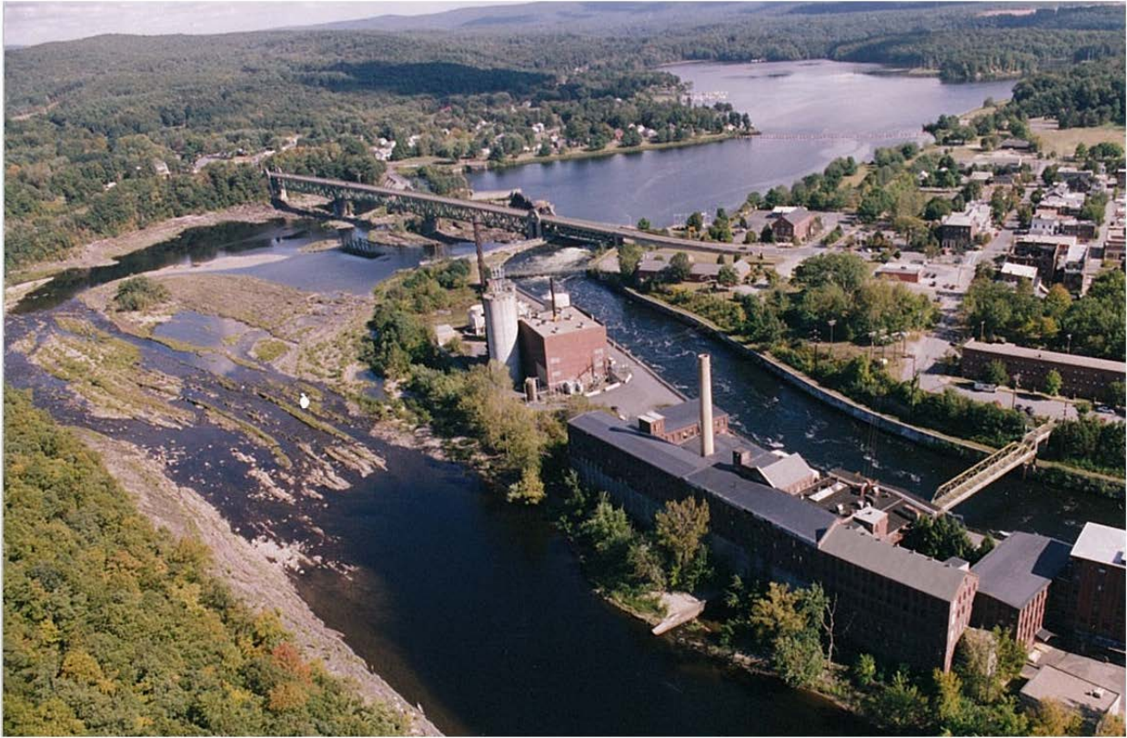
Figure 4.9.2-3: Aerial View of Turners Falls Dam Area, Looking Upstream
