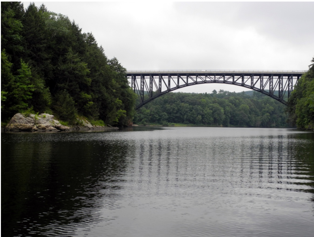
Figure 4.9.2-2: French King Bridge over Turners Falls Impoundment
