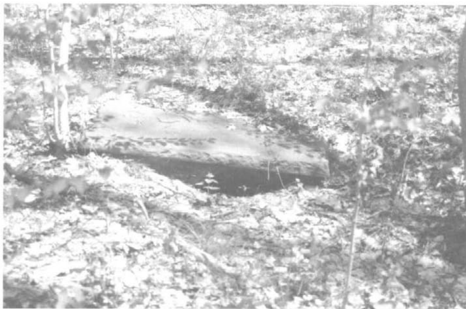
FIGURE 4.25: Culvert on south side of carriage road, 1993. (Photograph by author).
