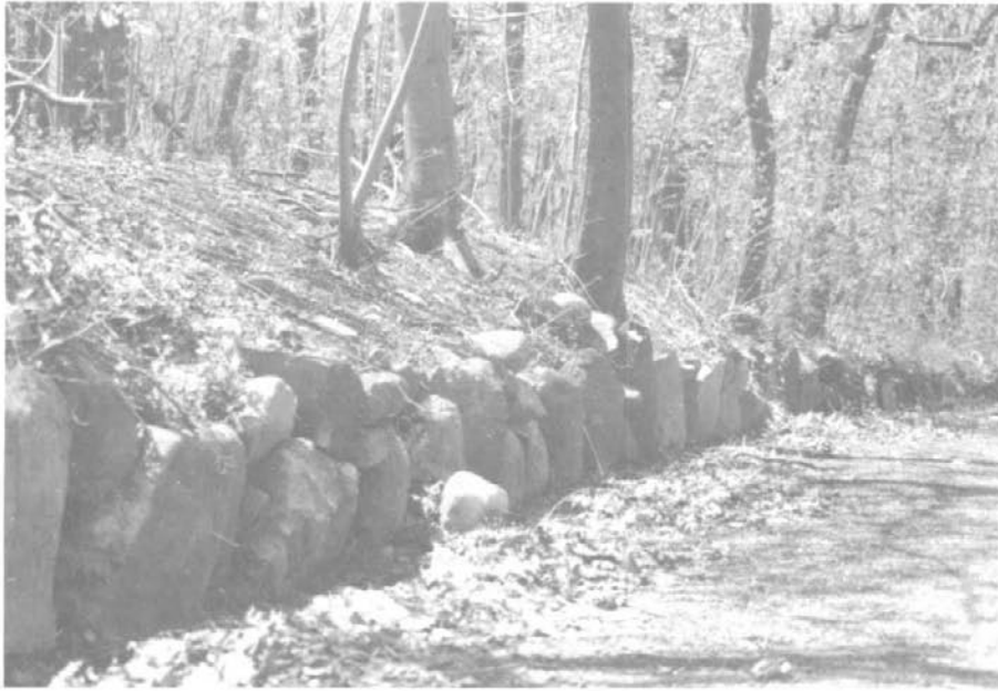
FIGURE 4.27: Dry-laid stone wall near entrance driveway, 1993. (Photograph by author).
