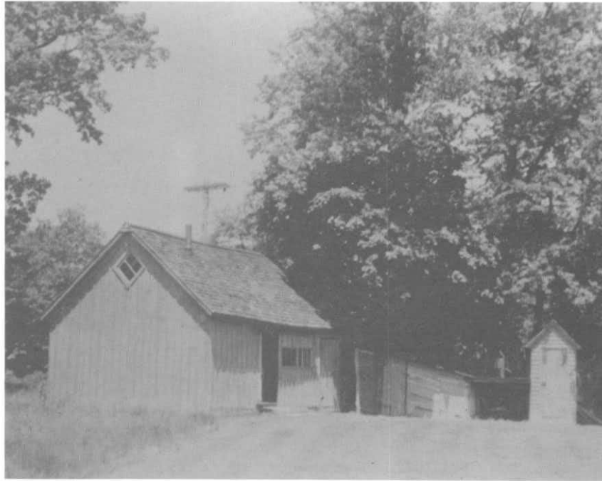
FIGURE 2.8: Sheds near Gardener's shed, 1950. (SAHINHS, TRA Materials, Box 5, Folder 2, GAIC "L").
