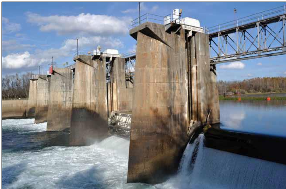
Figure 18: Downstream View of Dam and Gates, Facing Northeast (December 2012)
