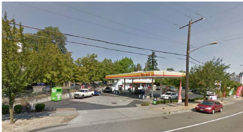
F. Shell Gas Station & Convenience Store
