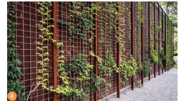
Greenscreen (at retaining walls only)
