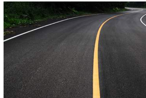
3. Asphalt drive aisle
