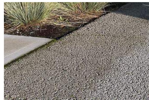
4. Permeable concrete sidewalks
