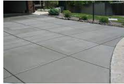
1. Scored concrete (motor courts and drive aisle crossings)
