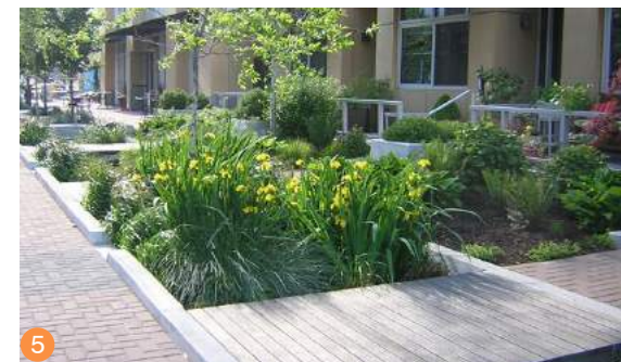
At-grade bioretention and pathway
