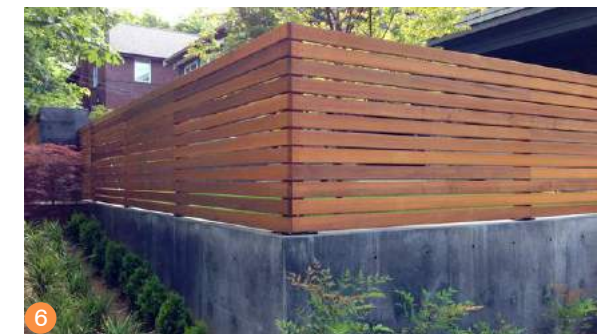
Wood Guardrail / Fencing
