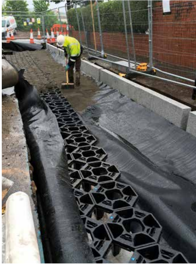
▲ Installation and completed works at Greener Grangetown. (© ARUP).
